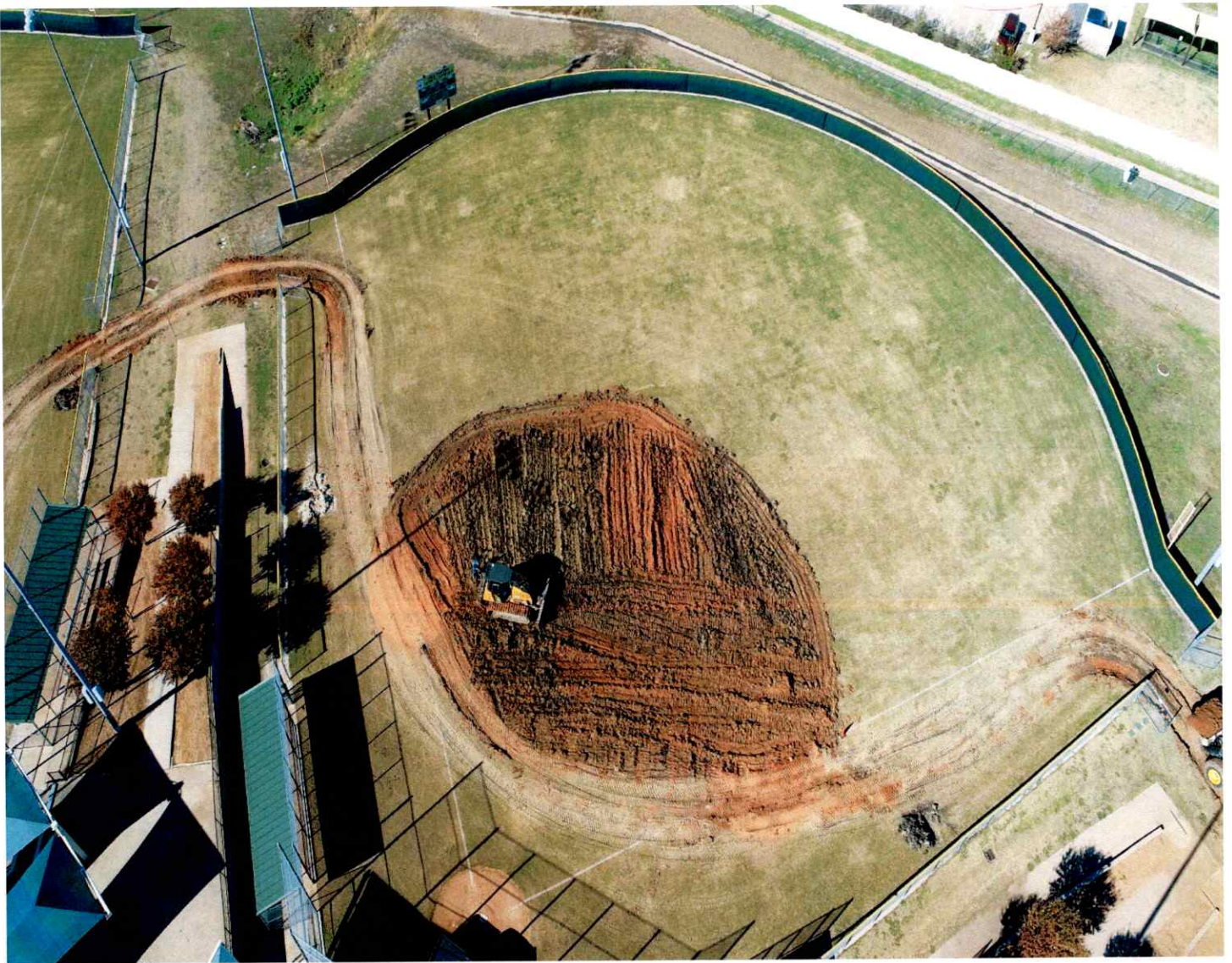
Synthetic Turf Improvements PH4 Field #9 – Dirt excavation
