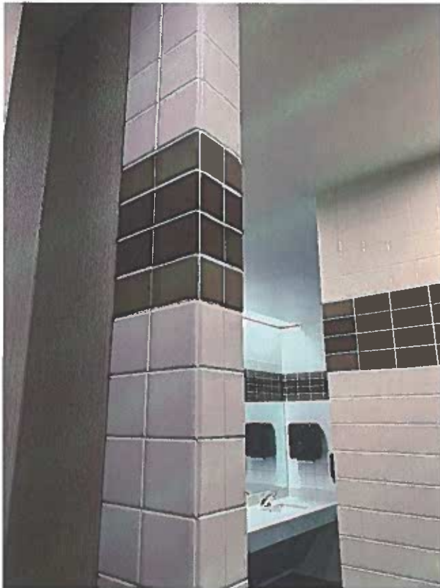
Restroom Change Order Item (Bull Nose Tile/Completed): Photo taken by WCC Staff
